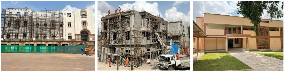
First Lady and Minister of Education and Sports, Hon. Janet Kataaha Museveni Lays Foundation Stone for the Reconstruction of the Main Building, 17th May, 2022
